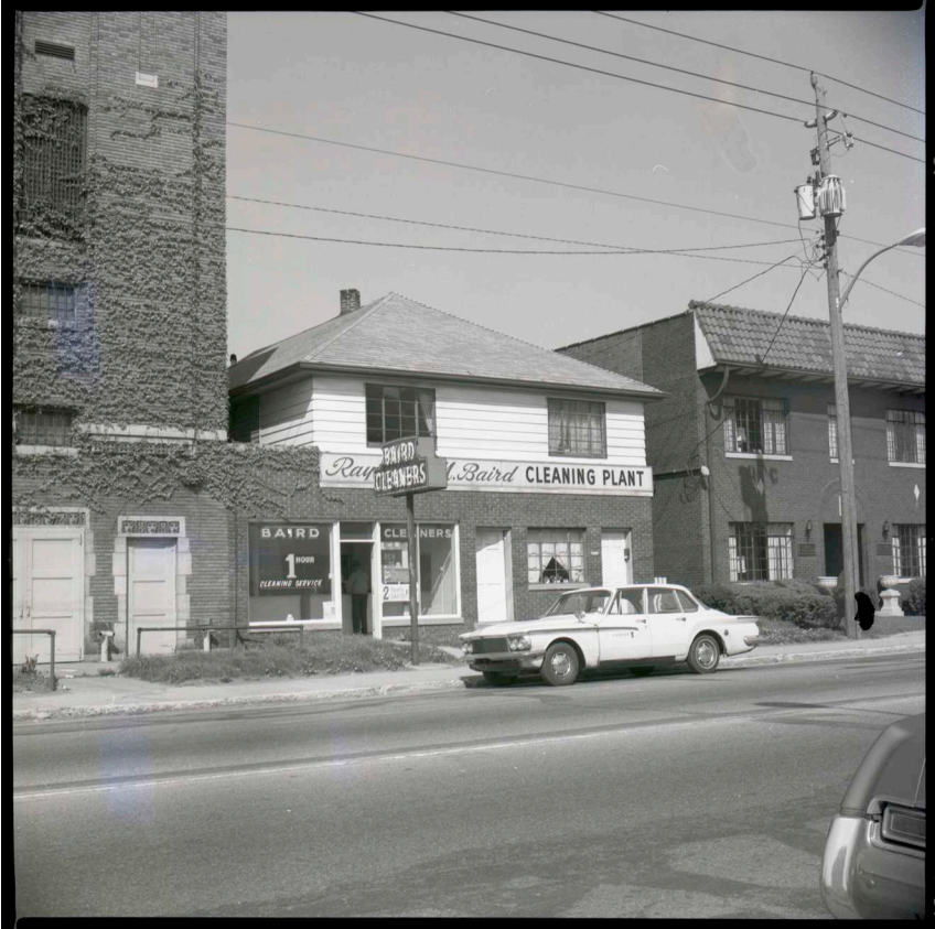
FIGURE 13.4 Baird Cleaners, 628 West Street, Indianapolis, c.1975. (Indiana Landmarks).
