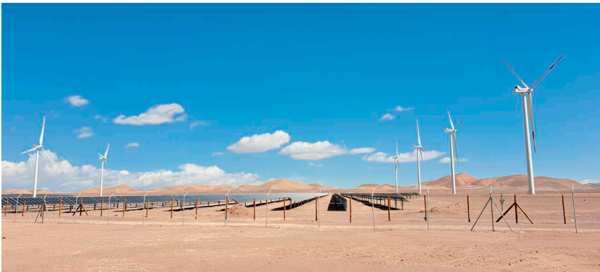
FIGURE 7.4 Solar panels of a wind turbine generator, by the authors.
